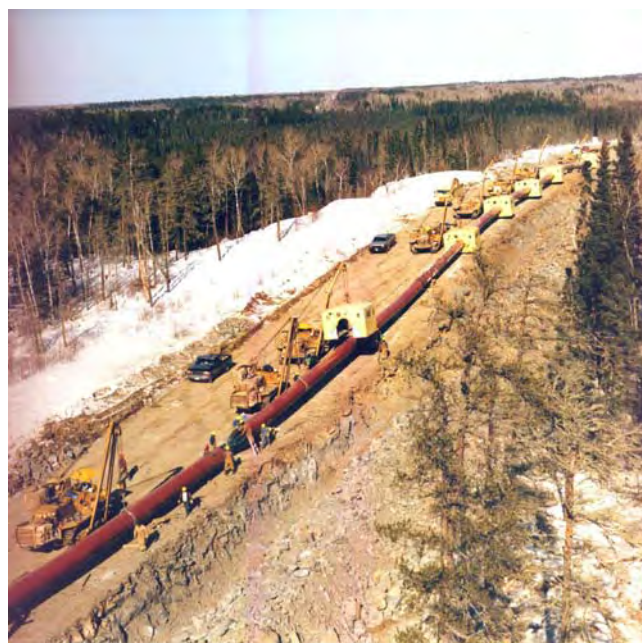
Figure 1: Welding sequence during pipeline construction
